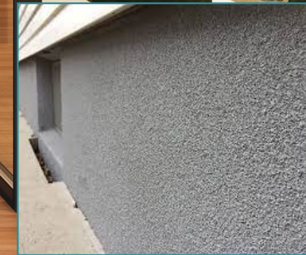
Thermal Protection Roof & Walls
